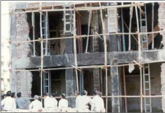
← Plate 9: Structural Repairs in progress
