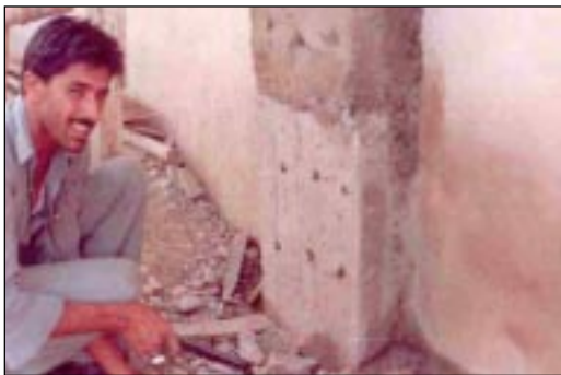
← Plate 5 : Injection Grouting
