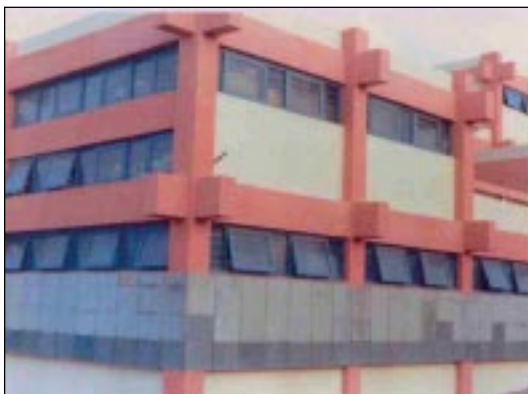
← Plate 7 : Building after rehabilitation
