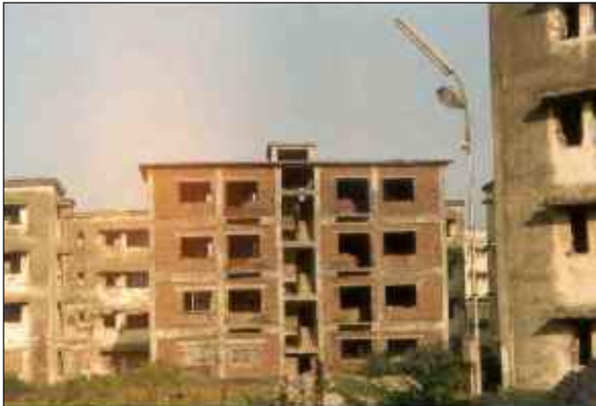
← Plate 10: Structurally repaired block before finishing before finishing
