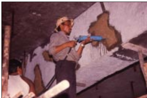
← Plate 6 : Injection grouting in progres.
