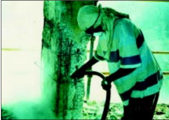
← Plate 10: Chipped Column with exposed reinforcement being cleaned by sand blasting
