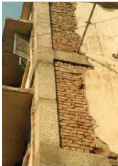
← Plate 8: Repaired column
