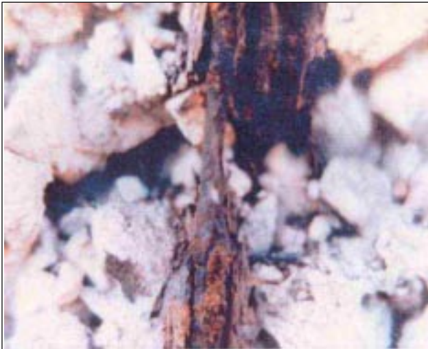
← Plate 2 : Rusting of reinforcement
