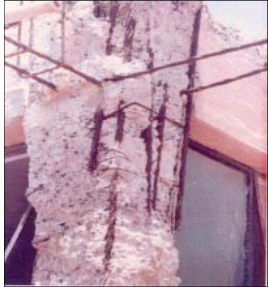
← Plate 2 : Rusting of reinforcement
