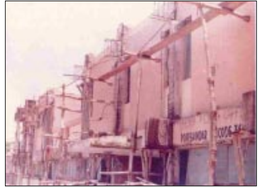
Plate 4 : Rehabilitation work in progress →
