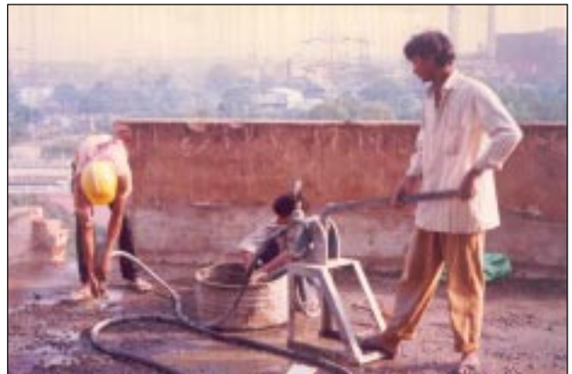
Plate 16: Cement Grouting in Honey Combed Concrete →
