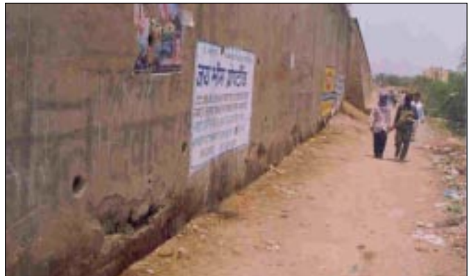
Plate 4: Damage due to urination near ground level of Counter-fort Retaining Wall →
