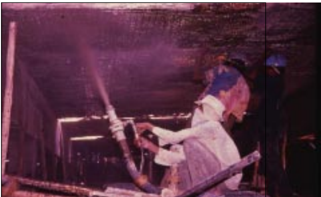
Plate 8 :Shotcreting in progress.
