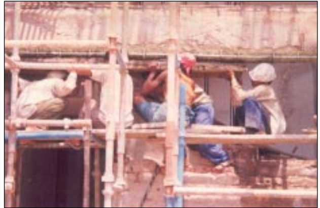
Plate 14: Repair material application to Soffit of RCC Beam →
