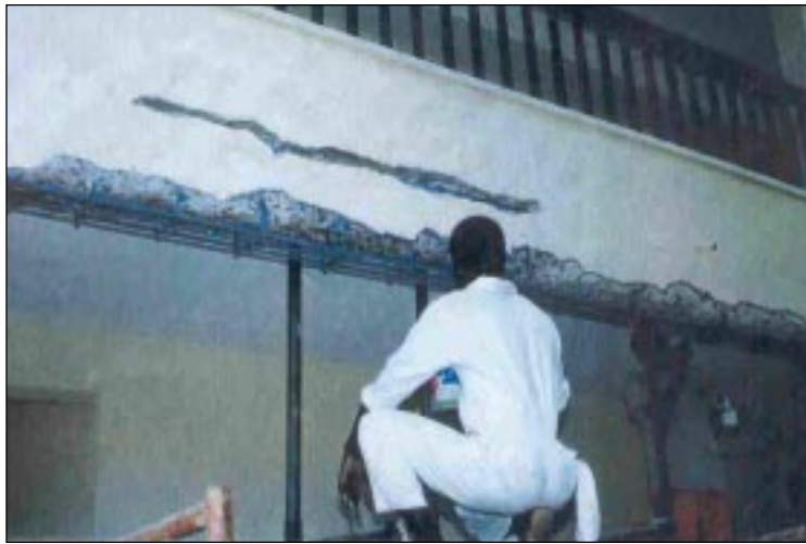
Plate 1: Rehabilitation work in progress.
