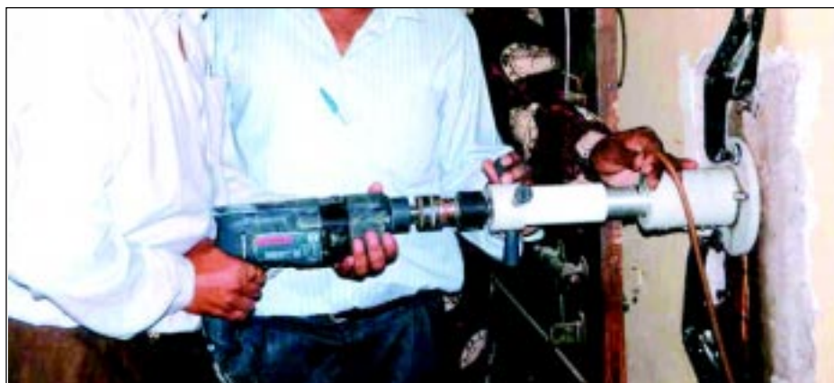
Instrument showing core cutting
