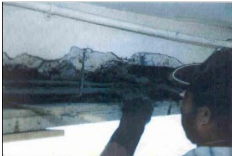
Plate 2: Rehabilitation work of beam in progress.
