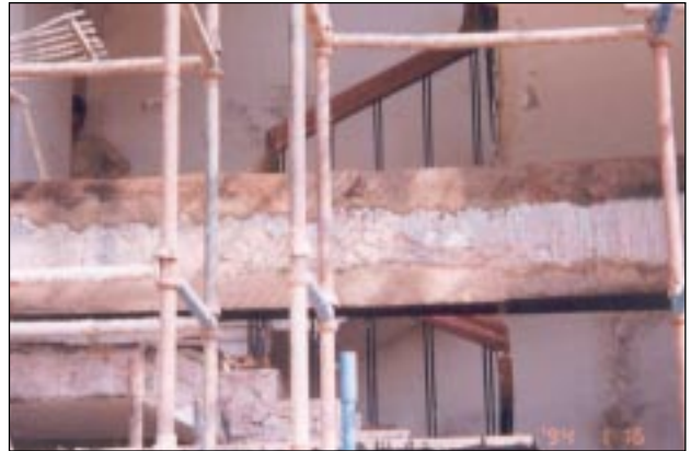
Plate 15: Repaired Beam →
