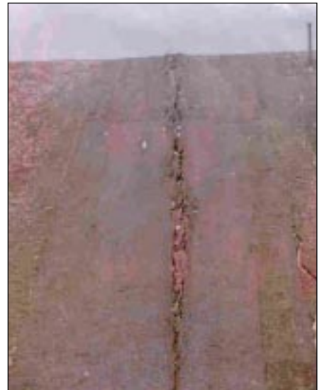
Plate 3: Expansion Joint as provided originally. The outlived tarfelt visible.
