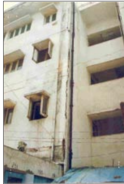
← Plate 6: Spalled cover concrete and exposed corroded reinforcement
