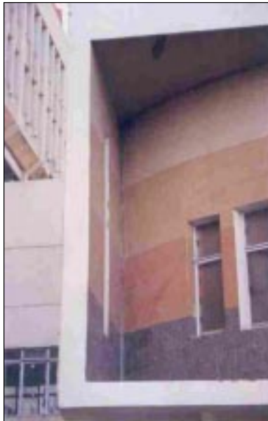
← Plate 2: Separation gap between the curved wall and the straight wall
