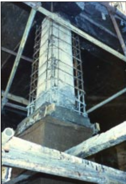
← Plate 4: Column Jacketting.
