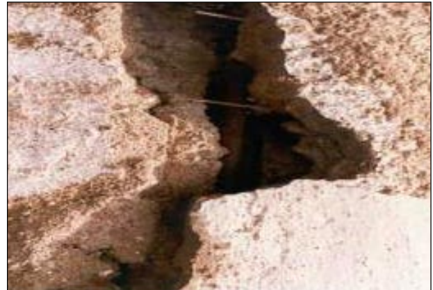
← Plate 4: Reduction of clear bay width due to increased volume of corroded reinforcement of RCC columns causing compression of balcony railing
