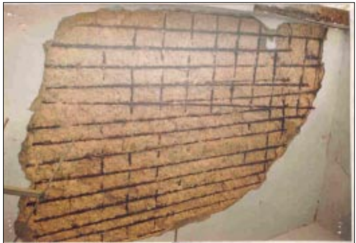
Plate 7: Spalled Cover Concrete of RCC Slab →
