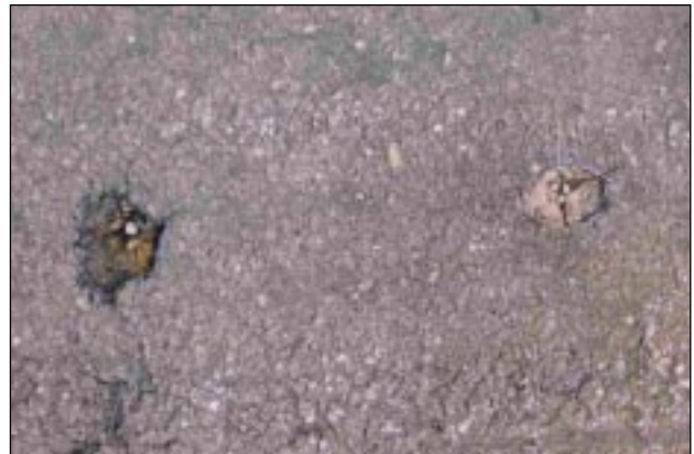
Plate 3: Expansion Joint as provided originally. The outlived tarfelt visible.
