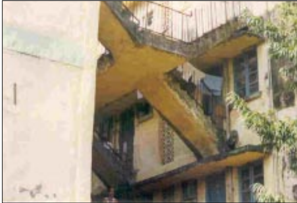
Plate 3: Earlier repaired Column Damaged → again due to corrosion
