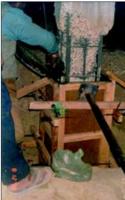
← Plate 12: Micro-concreting being done to RCC jacket
