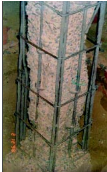
Plate 11: Exposed reinforcement and chipped concrete after sand blasting →
