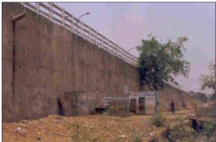
Plate 1: General View of the Counter-fort Retaining Wall →
