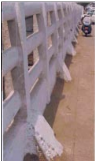
Plate 4: Damage due to urination near ground level of Counter-fort Retaining Wall →
