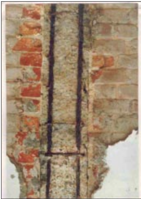
← Plate 6: Spalled cover concrete and exposed corroded reinforcement
